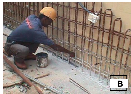
Photos A & B: Applicator is applying Everdure Adhesive before installing EVERDURE WATERSTOP RTD series in position.
