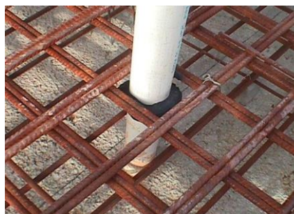
Photos A & B: Applicator is applying Everdure Adhesive before installing EVERDURE WATERSTOP RTD series in position.
